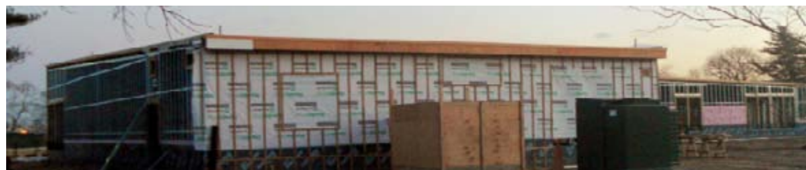
New Children's Center to open near the Route 110 entrance
